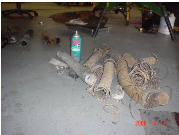
Worn Ventilation Ducting
