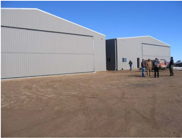
Pictured above are the fronts of both hangars. The hangar with the smaller door is to the east, and will house the snack bar, store, and achieves and reading room.
